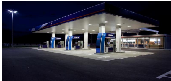
Gas station Ina Karlovac
