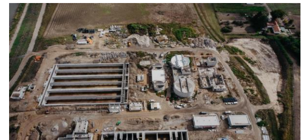
Wastewater treatment plant Osijek
